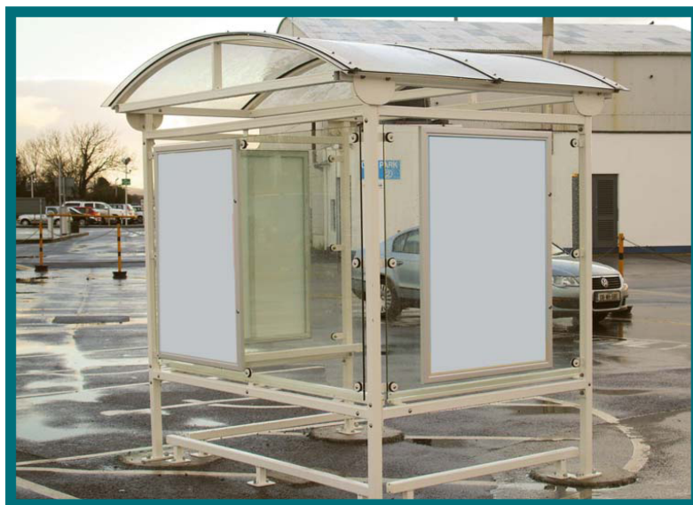
On the sides of trolley bay in car park
